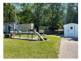
These 4 wells operate around the clock on a rotating demand system and ramp up as demand increases. Collectively they are able to pump over 6,000 gallons per minute if demanded. In recent years, they have been modernized with new energy efficient pumps and control systems saving our customers 20-30% in operating costs. These critical well stations are monitored 24 hours a day and
